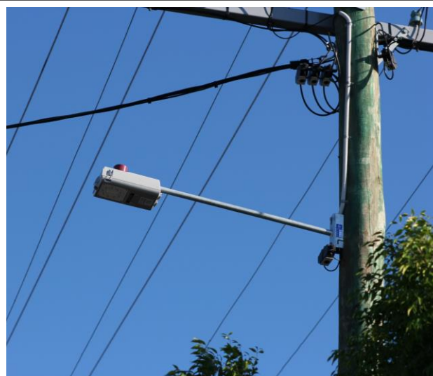
None of the trial luminaires in this street have been installed horizontal.
