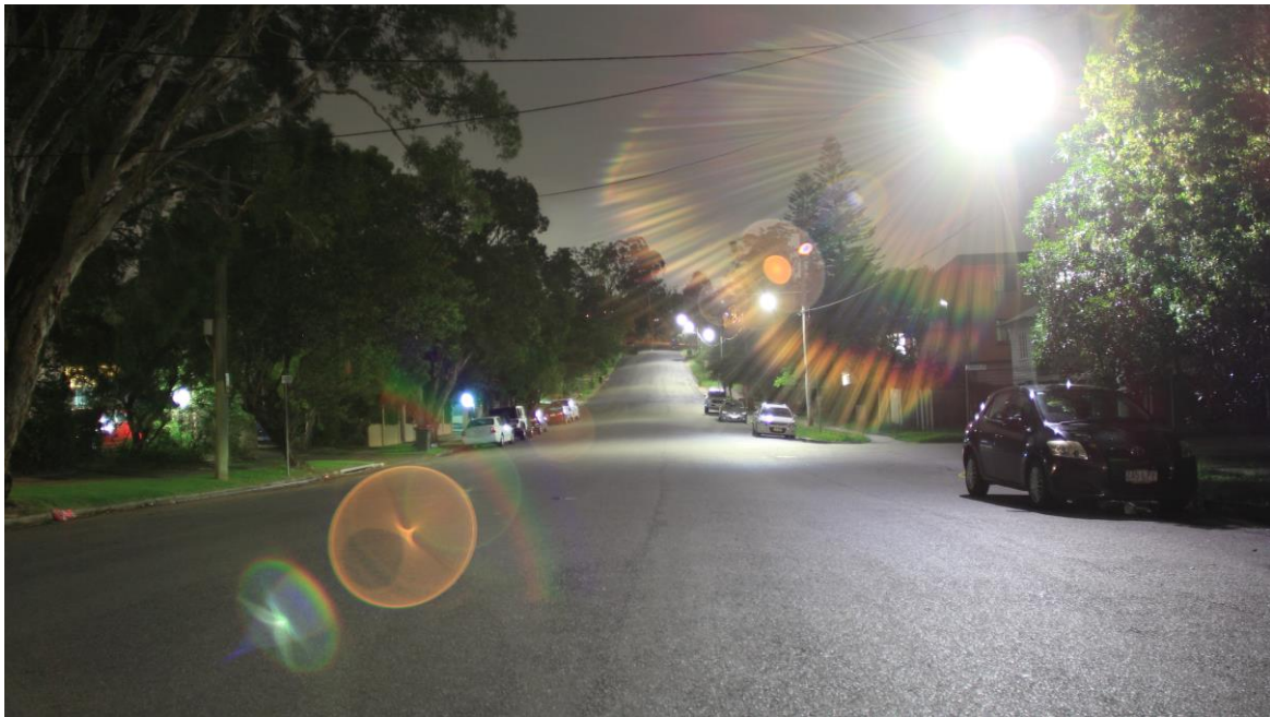
These luminaires cast a very extensive illumination pattern with very bright regions below each pole.
