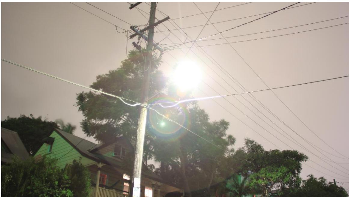
This luminaire is very glary for pedestrians and causes significant light trespass.
