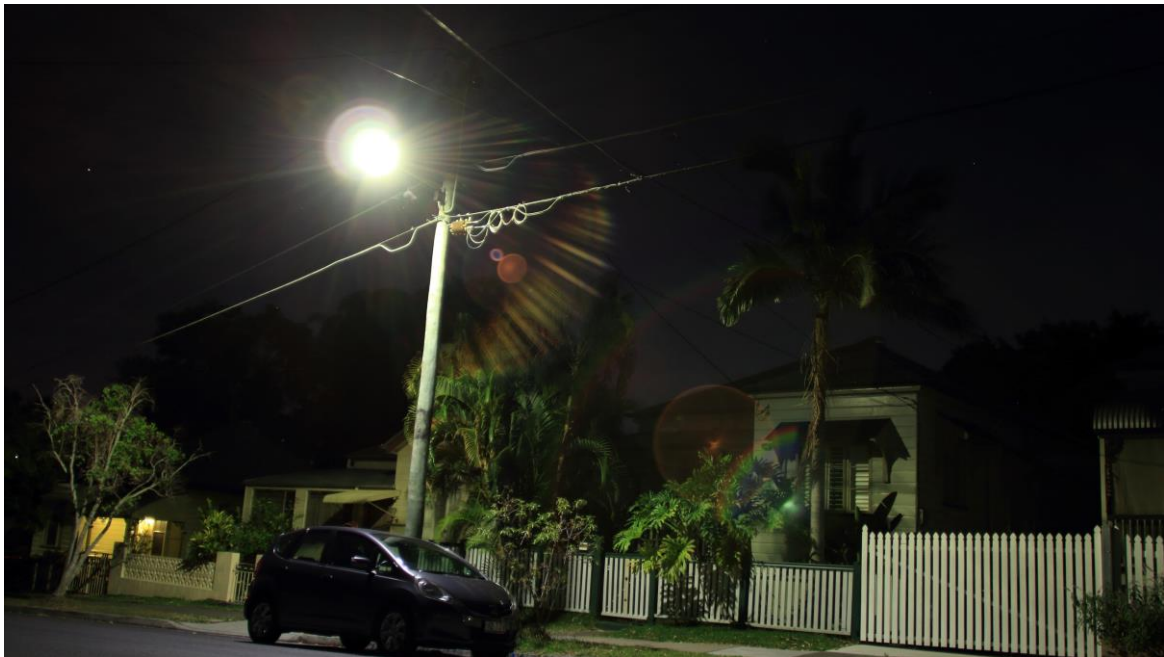
Significant rear light trespass into homes.
