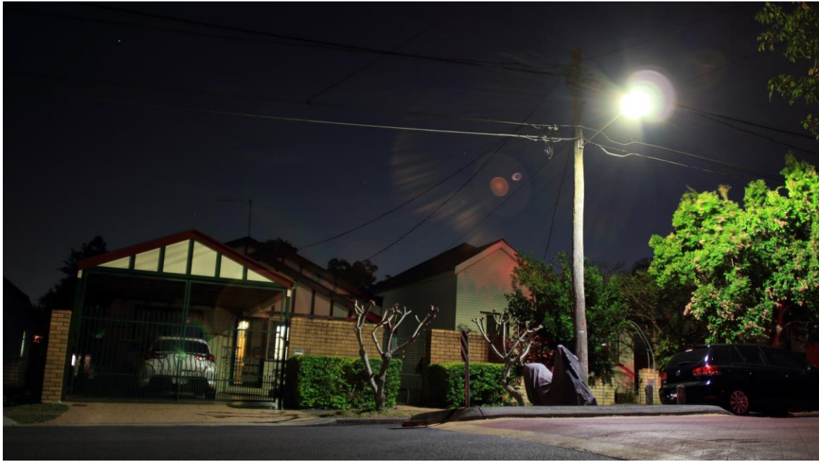
Significant rear light trespass problem with this luminaire.
