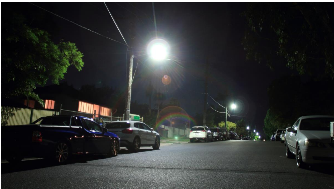
This luminaire is intensely glary and projects trespass light to the rear.
