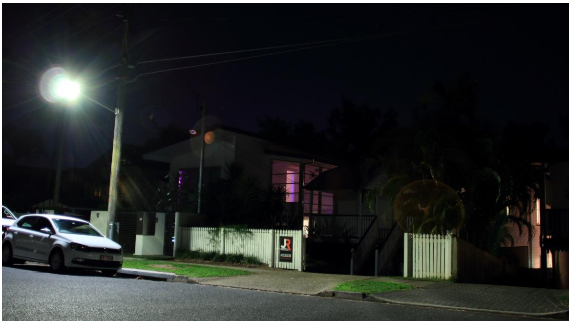
This luminaire is intensely glary and projects trespass light to the rear.
