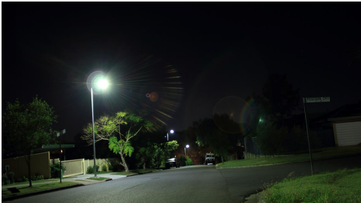
Forward light extends across the roadway and may annoy residents on the opposite side of the street.
