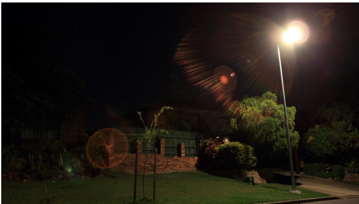
An example of backward light trespass onto private property – western end of Galleon Street, Jamboree Heights.
