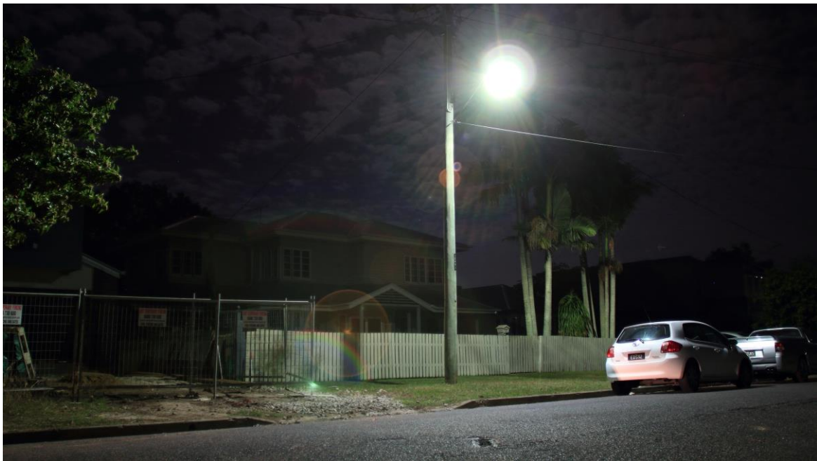
This luminaire is intensely glary and creates too much light trespass to the rear.
