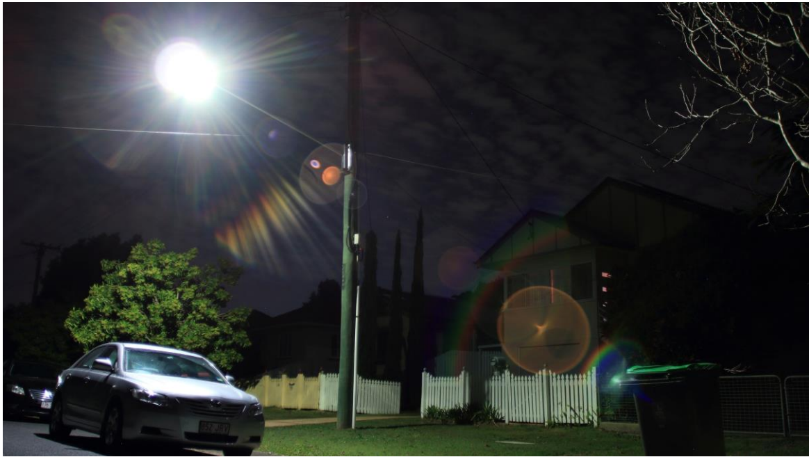
This luminaire is intensely glary and creates too much light trespass to the rear.
