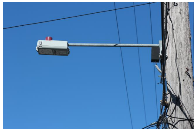
All the trial luminaires have been installed with an up-tilt angle of at least a few degrees.
