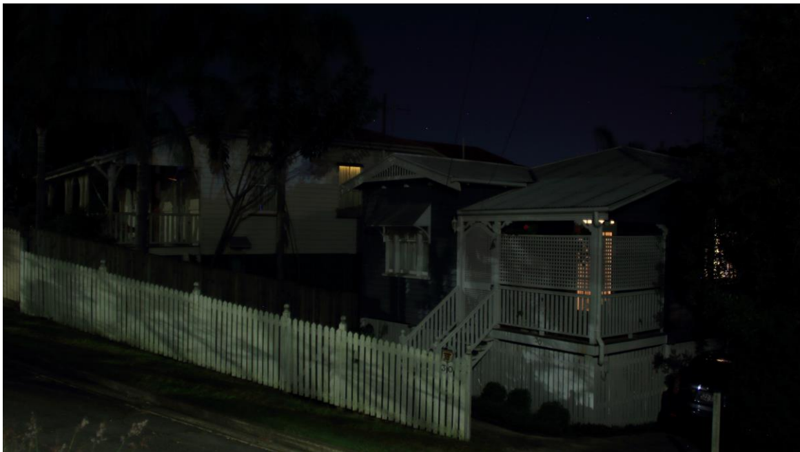
This luminaire projects light trespass and glare far forward and into properties across the street and far from the luminaire.
