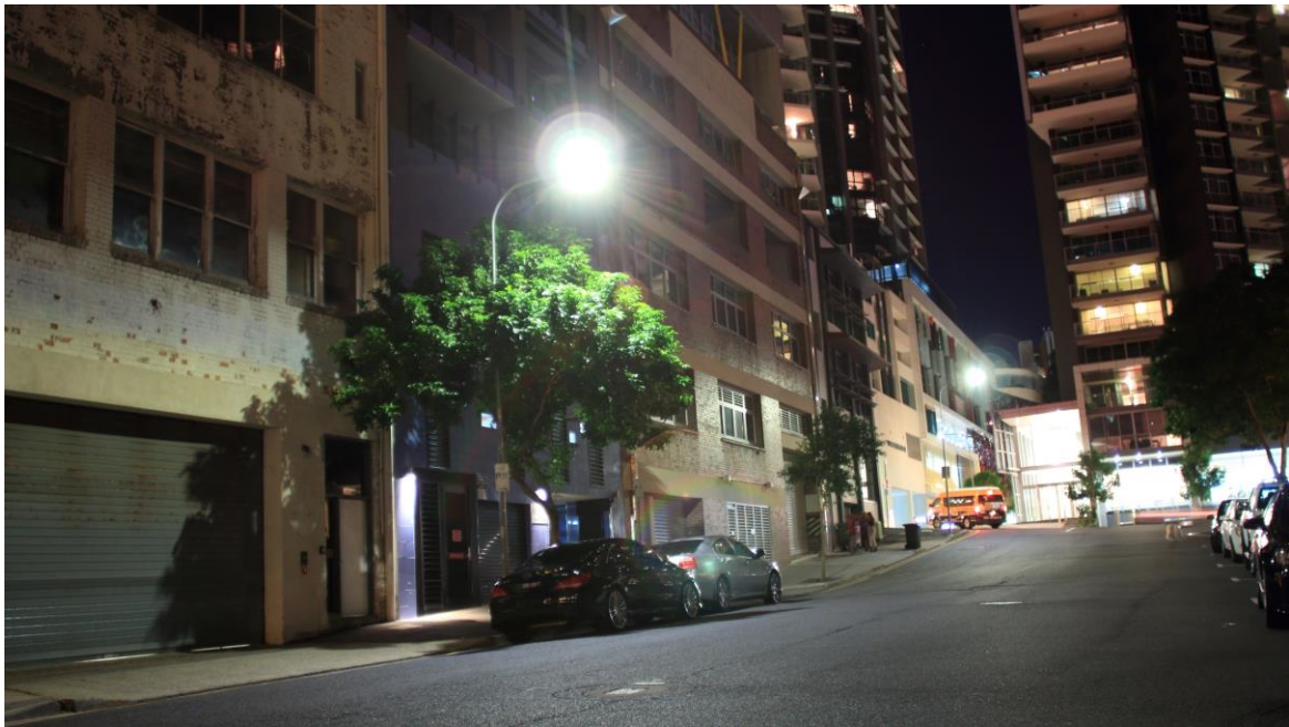
These luminaires are very bright and excessively glary for use in residential streets.
