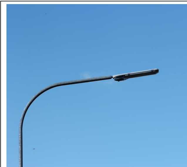
All these trial luminaires have been installed with a significant up-tilt angle, some excessively so.
