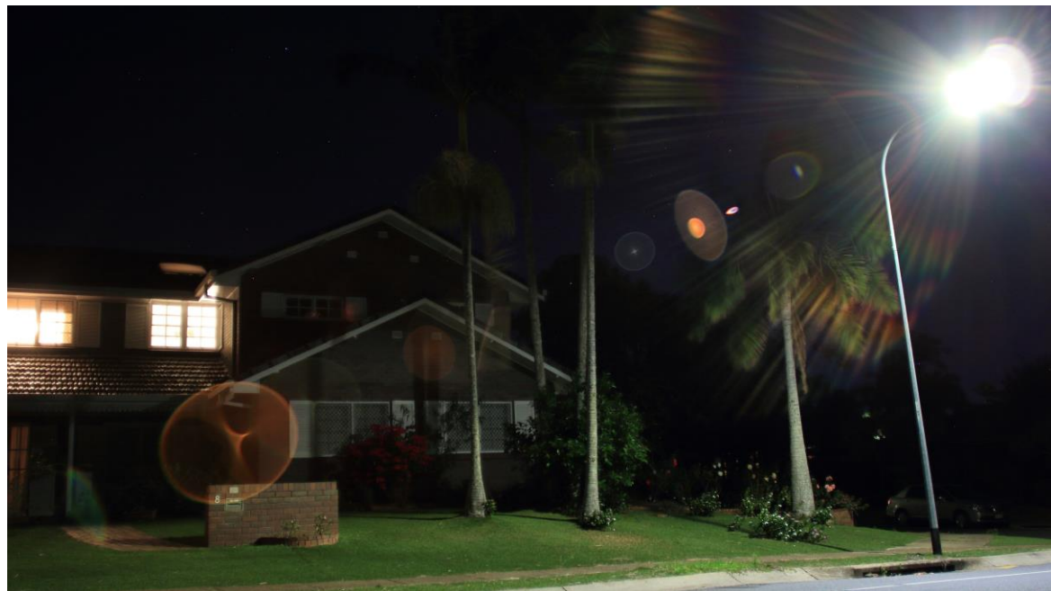
This luminaire projects considerable trespass light to the rear on to private properties. It is also excessively bright and glary for residential streets.
