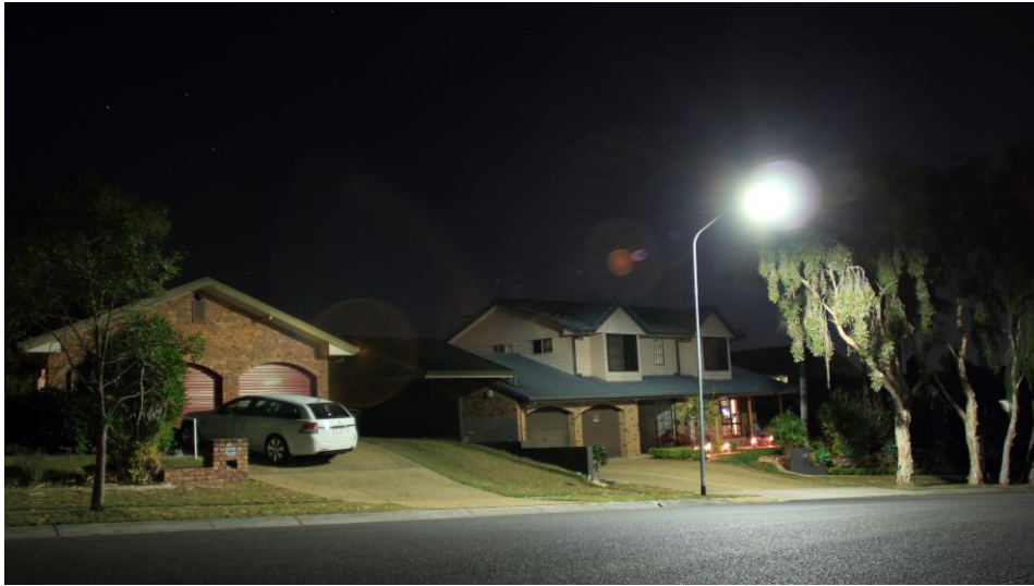
Malbon street – west. Excessive rear light trespass.
