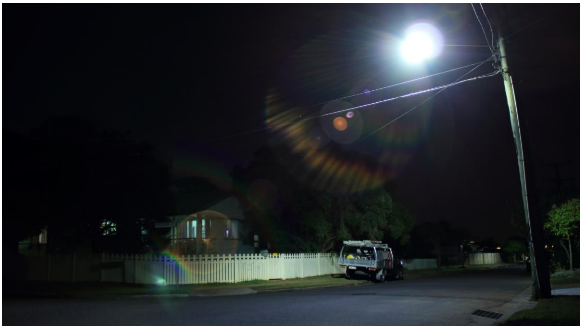
Substantial forward light trespass and glare zone nuisance light on to private properties.
