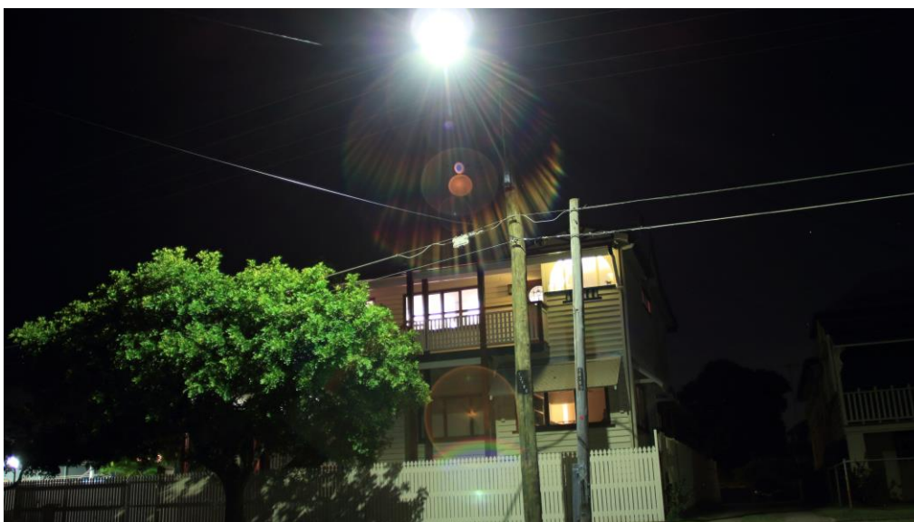
Excessive rear light trespass.
