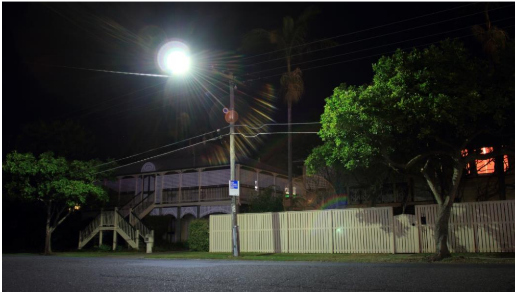
Poor control of rear trespass light onto private property.
