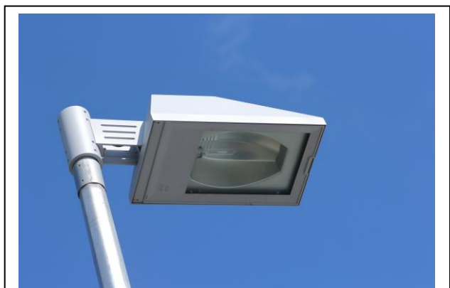
Shielded carpark luminaire on private property on Third Avenue, Sandgate.
