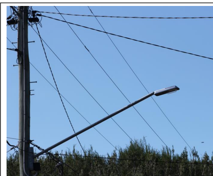
Trial luminaire installed with an up-tilt angle estimated at 17°.
