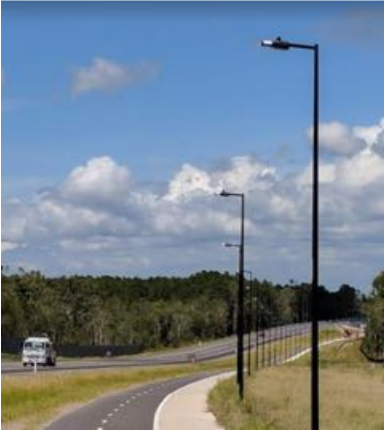
Figure 17. Queensland Department of Main Roads unshielded blue rich LED lights installed February 2017 on Caloundra South access road. (Author's Personal Photo)
