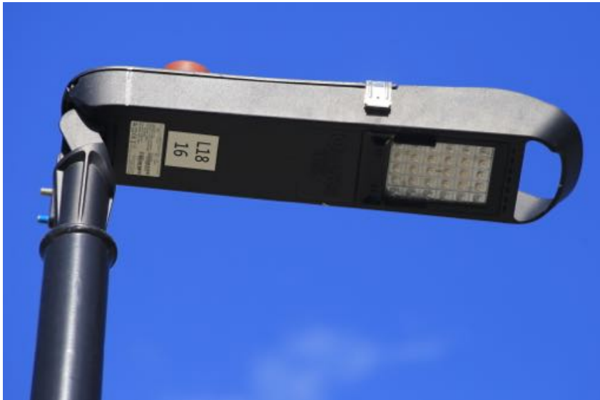
Figure 15. International Dark-Sky Association Compliant LED luminaire as used in the Sunshine Coast Urban Lighting Master Plan. (Author's Personal Photo)
