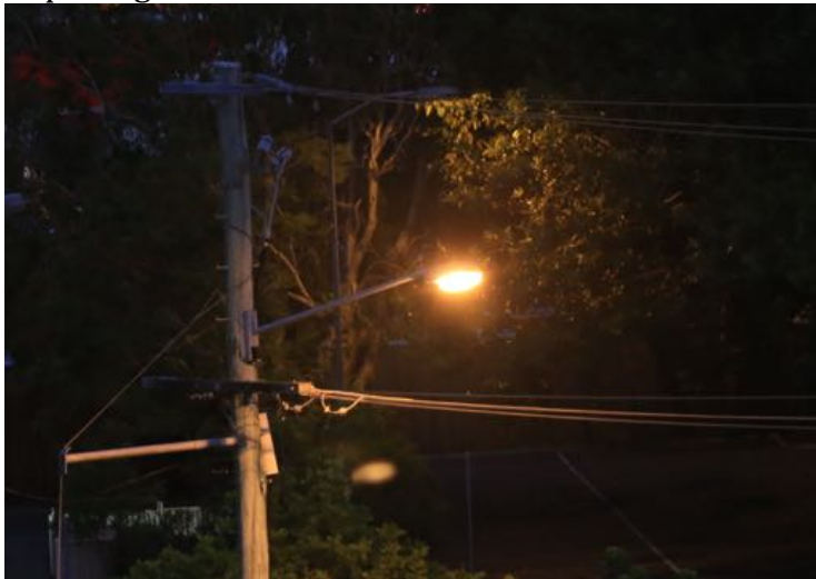
Figure 14. Unshielded high pressure Sodium Luminaire from 5 degrees above horizontal (Author's Personal Photo).
