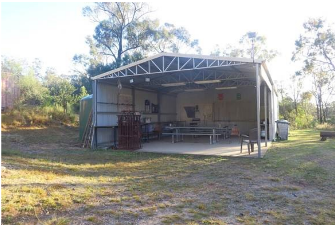
The WDA main shed. The northern half is lock-up while the southern half is open area and has the refrigerator and microwave etc.
