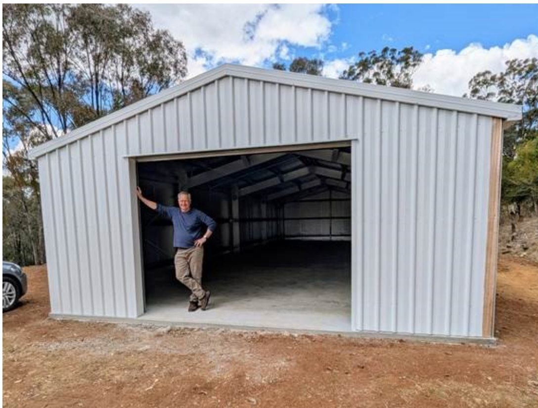
6mx15m steel shed, insulated. (Please do not drive vehicles into the shed.)
