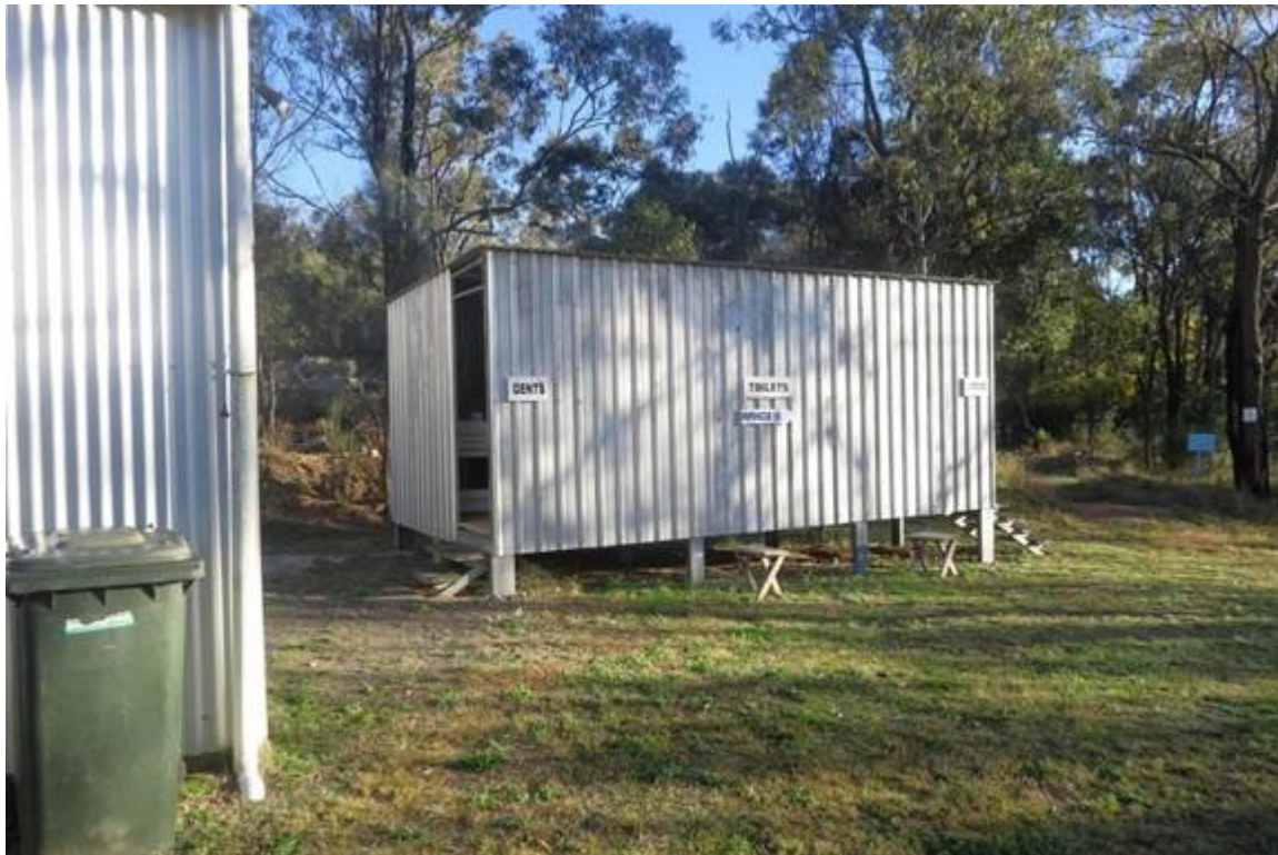
Archers' toilet and shower facilities
